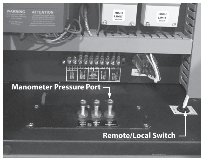
Figure 22 Manometer connections to manifold
